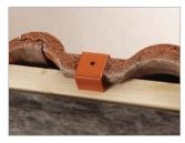
2. Fitting to each roof tile insert the snowstop hook centred into the headlap part of the tile.
