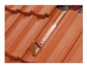
3. The roof tile above is also laid on the roof's surface so that the snowstop hook is inserted securely in the headlap joint.
