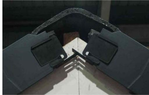
6. Insert a Ridge Closure into the last Unit, interlocking the combs of each Contract Dry Verge Unit at the apex.
