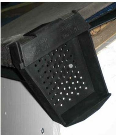
2. Fix the Eaves Closure to the end of the fascia board or brickwork.
