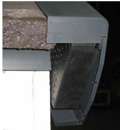
3. Fit the first verge section ensuring that it is located onto the eaves closer.
