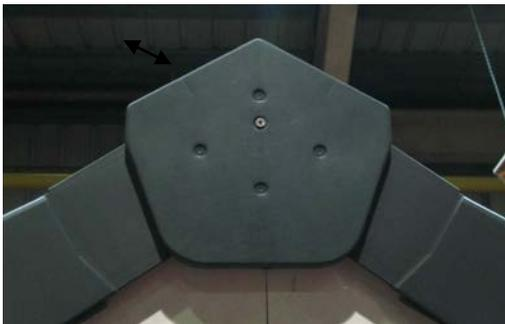
7. Screw fix the Ridge End Cap to the ridge batten.
