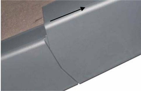
5b. As each successive verge tile is laid, slide on a Contract Dry Verge Unit up to the tile toe, engaging with the Unit below, nail in position through the Batten End Clip into the batten.
