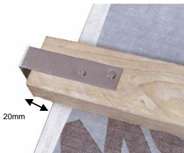
1a. Extend the tiling battens 20mm beyond the gable wall or barge board and nail a Batten End Clip to the end of every batten.
