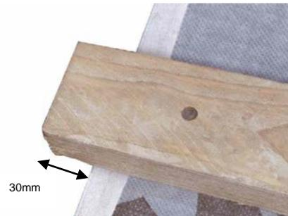
1b. If a batten end clip is not being used we recommend that the batten is extended 30mm over the barge board or brickwork and 40mm (minimum) x 3.25mm ring shank nails are used to fix the verge units. Prior to fixing the batten, ends must be in good condition with no signs of decay or splitting.
