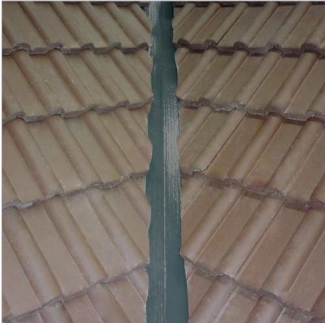
GRP Valleys provide a robust, durable and lightweight alternative to lead and zinc valleys.
