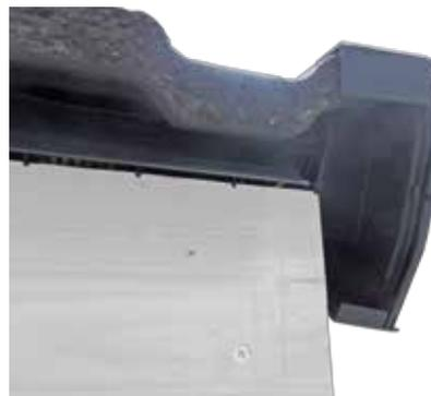
3. Fit the first verge section ensuring that it is located onto the eaves closer.
