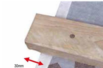
1b. If a batten end clip is not being used we recommend that the batten is extended 30mm over the barge board or brickwork and flat head screws are used to fix the verge units. Prior to fixing the batten, ends must be in good condition with no signs of decay or splitting.
