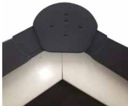
8. Screw fix the Ridge End Cap to the ridge batten.
