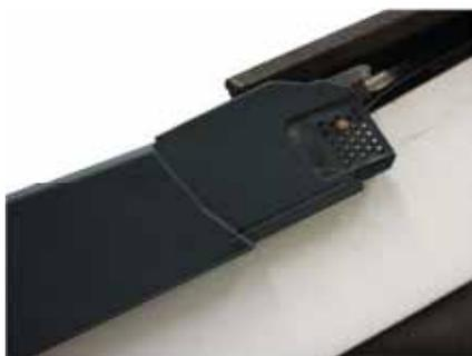
4. Nail in position, through the Batten End Clip into the batten.
