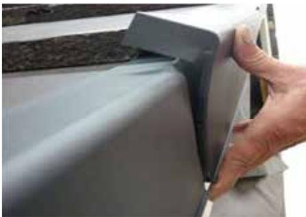
5a. Clip the bottom of the verge unit in place first, then lift the top of the verge unit over and clip in to place. As illustrated in stages 5,5a and 5b.
