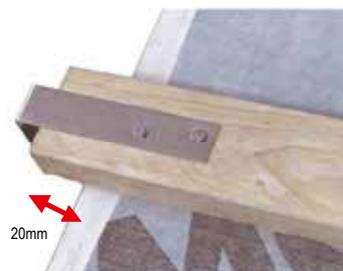
1a. Extend the tiling battens 20mm beyond the gable wall or barge board and nail a Batten End Clip to the end of every batten.
