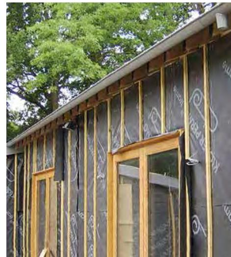
**Typical timber frame wall construction**
