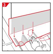
Remove protective film from the lower section and press onto the high points of profiled tiles. The EasyForm can now be dressed firmly into the pan of the tile, using a roller if necessary.
